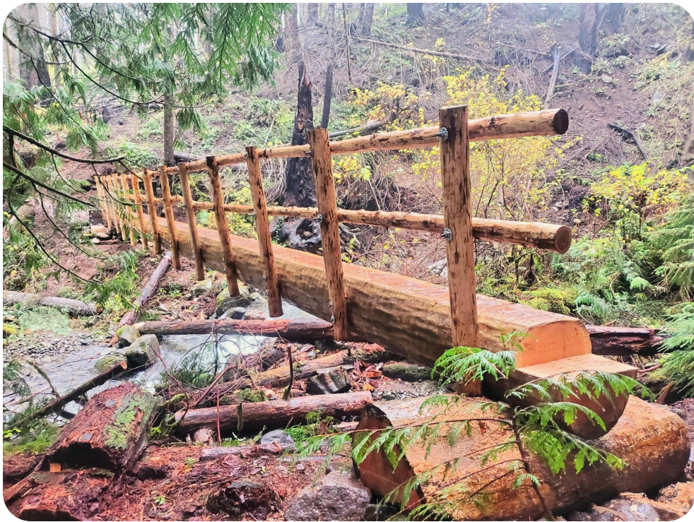
New Larch Mountain Trail Bridge (by USFS)
