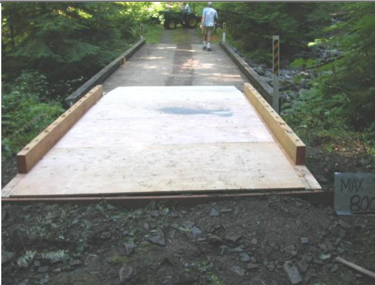
The Nesika temporary bridge ramp at Multnomah Creek by Randy Dietrich
