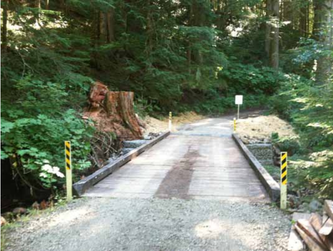
Completed Repair By George Milne
