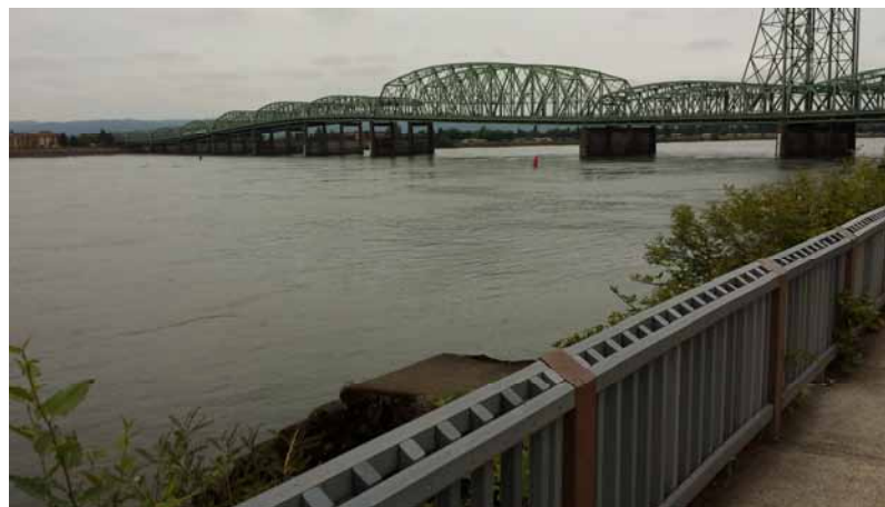
I-5 Columbia River Bridge By Phillip Jackson
