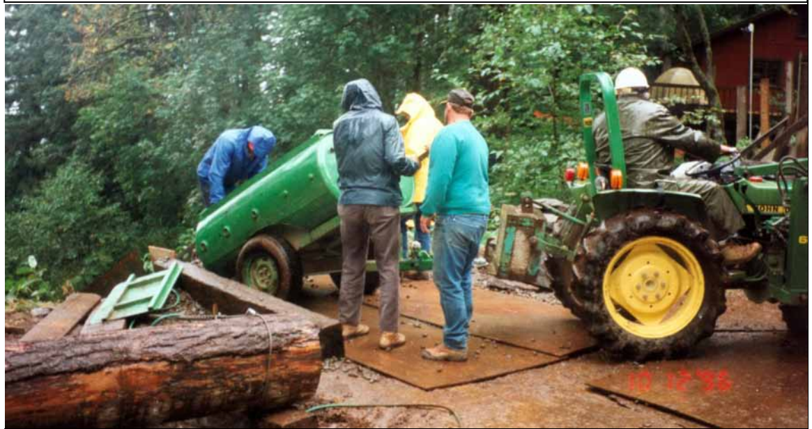
B Dump Trailer Used for Building Drainfield
